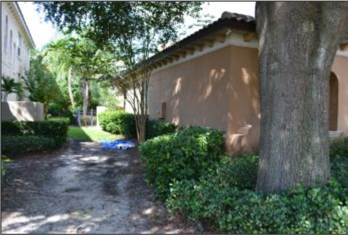
Left side of the home.
